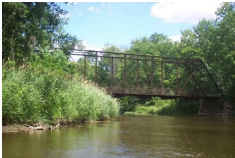
Six-Mile Creek 1886 Iron Bridge—restoration priority
