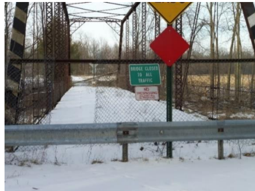
Restoration Site—Six Mile Creek Bridge
