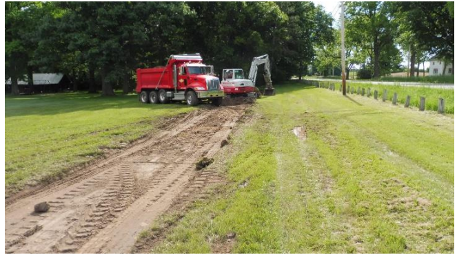
Constructing Henderson Loop Trail-2022
