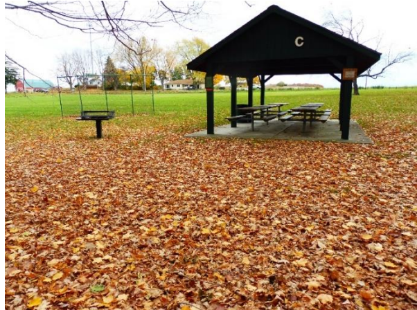
Henderson Park accessibility pathway need
